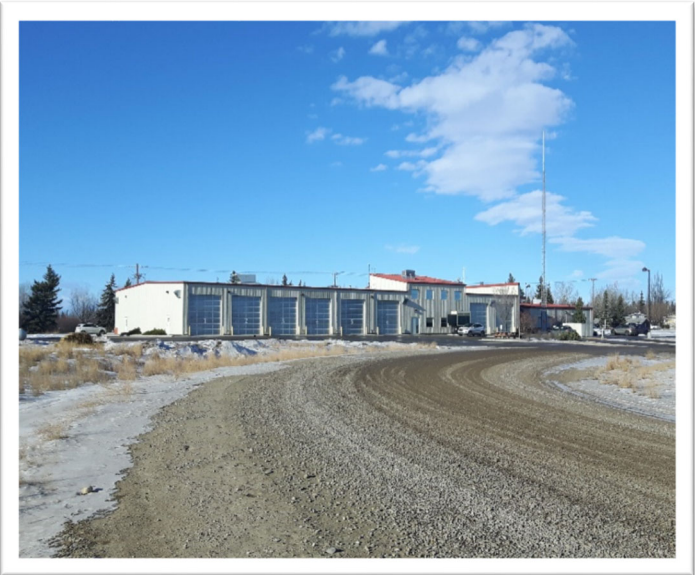
Looking northwest at the tri-services building
